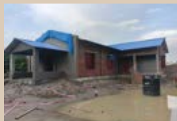
Rajshahi District church building project in progress
